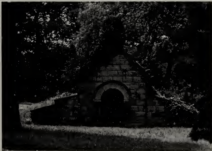
Receiving Vault where deceased may be placed awaiting interment.
